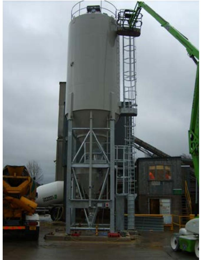
Vertical Cement Silo With Weigh Hopper
